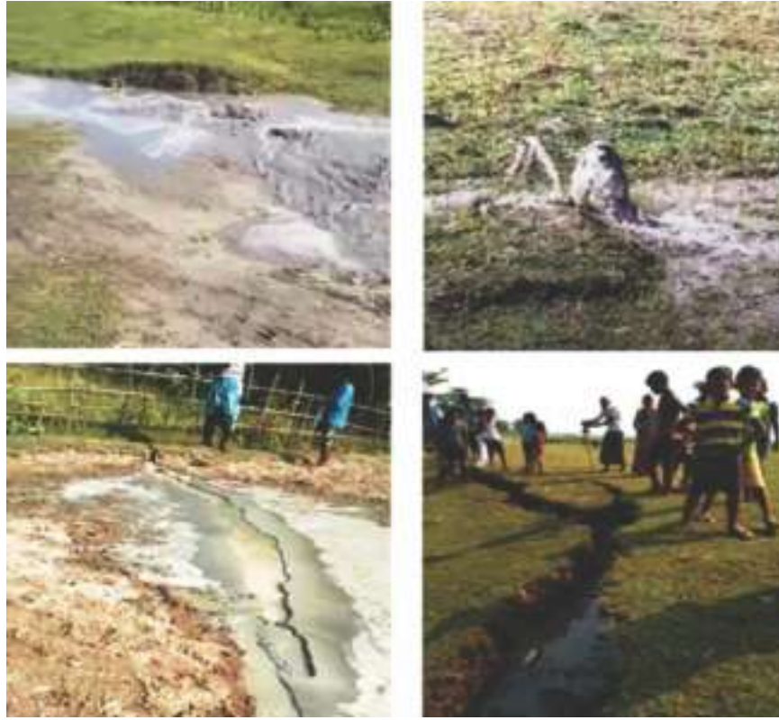
Fig. 3. Photographs of soil liquefaction in the form of sand dykes and sand boils along with ground cracks occurred aftermath of the 28 th April 2021 Dhekiajuli earthquake. The open ground crack image is collected from PTI, 28 th April, 2021.
